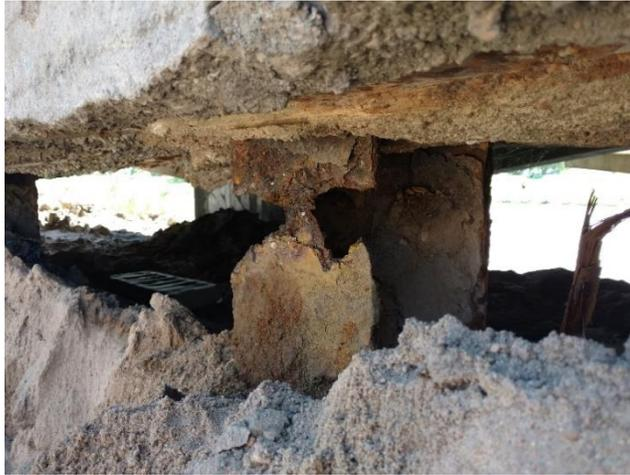
*Figure 1 – Corrosion of piles in deicing salt contaminated sand*
